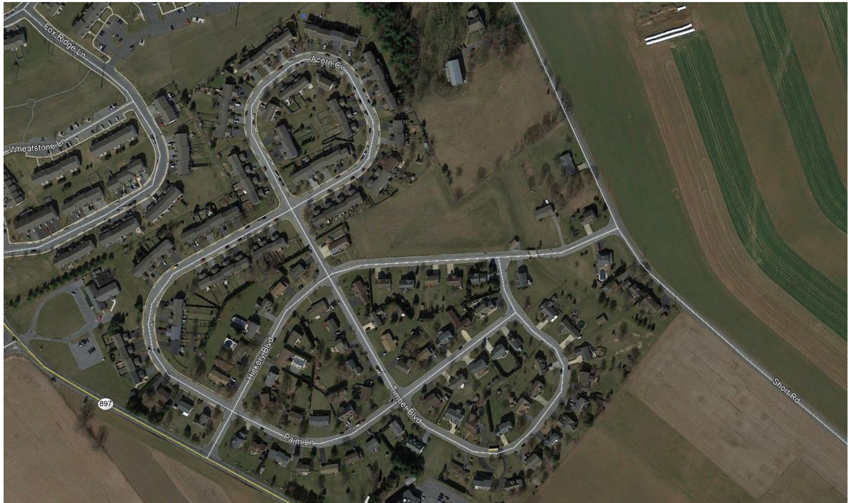
Hickory Boulevard Basin Retrofit Aerial Photo
