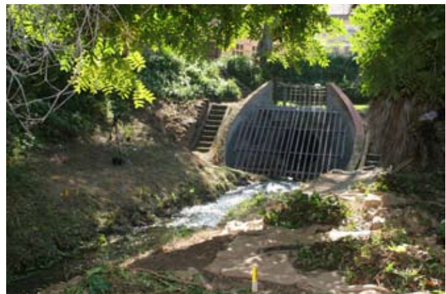
Figure 2–3 Daylighting stream project
