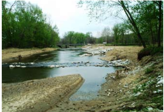
Figure 2-12 Local instability problem above a township bridge. This channel became misaligned with the bridge opening due to lateral migration. The treatment includes stream barbs and a rock riffle grade control structure to protect against possible degradation as a result of shortening the channel during realignment. (Bay Creek, Pike County, IL)
